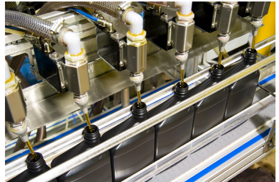
Figure 1. Valves in a Bottling Factory
