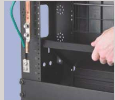
Bonding and grounding ready
