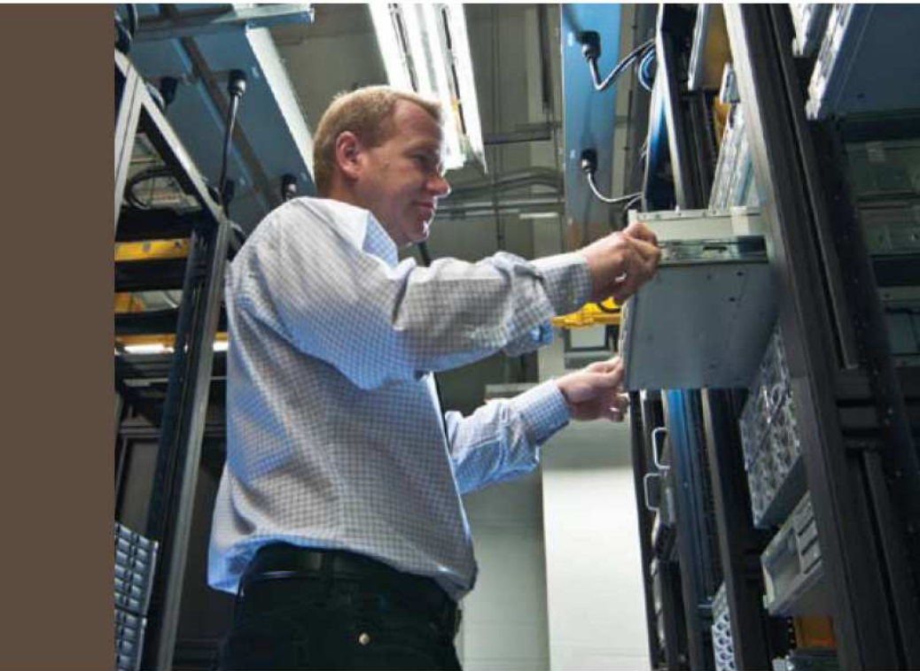
A 5 kW per cabinet hot-aisle/cold-aisle environment
