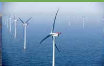
Wind power generation
