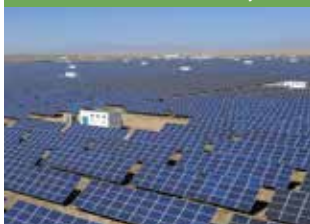
Photovoltaic Generation System
