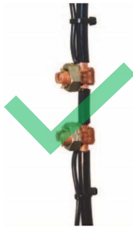
Figure 1 Example of properly terminated sensor leads. Lead are not mechanically connected and termination points are insulated.
