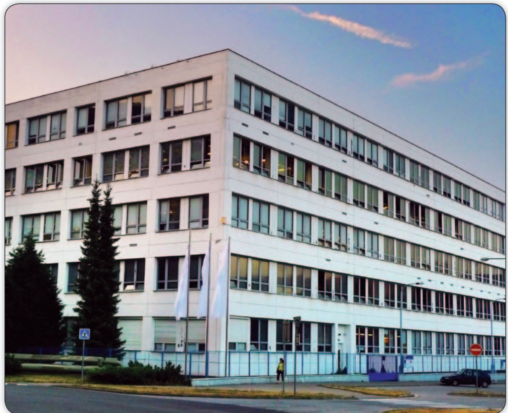
TE Manufacturing Facility in Trutnov, Czech Republic
