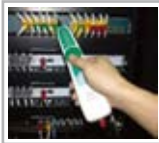
Copper cabling detecting, including shielded (STP) and UTP cable
